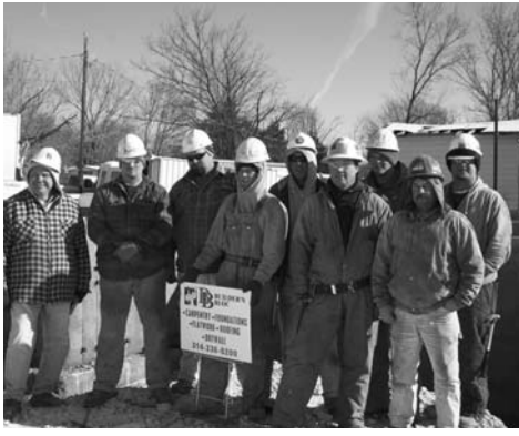
The crew from HBA associate member Builder's Bloc put in the foundation of the Hornbeck/Akers house.
